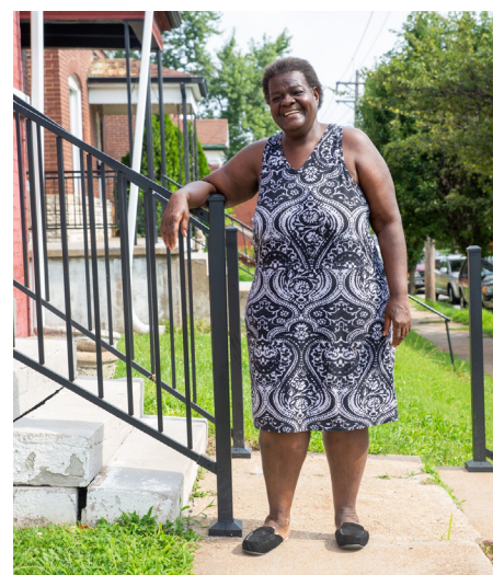
Mary Bobo, a client of Mission: St. Louis, had new handrails installed on her front steps by the Home Repair Team. Repairs and home modifications completed by the organization help area residents remain independent in their own homes. Photo: Colleen O'Connell Smyth, Mission: St. Louis.
